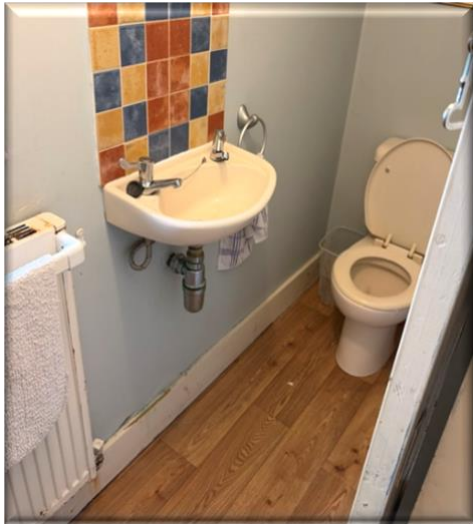
WC / Shower Room
